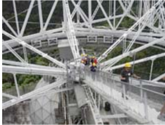
Figure 3: Azimuth hub with the Gregorian dome below.
