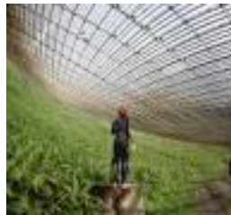
Figure 10: A view from down under.
